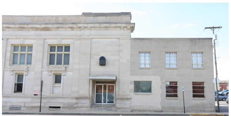
This historic bank has a rear addition for extra office space. The addition respects the historic building in scale and it's proportion of openings, and the style and character of a more modern design.
